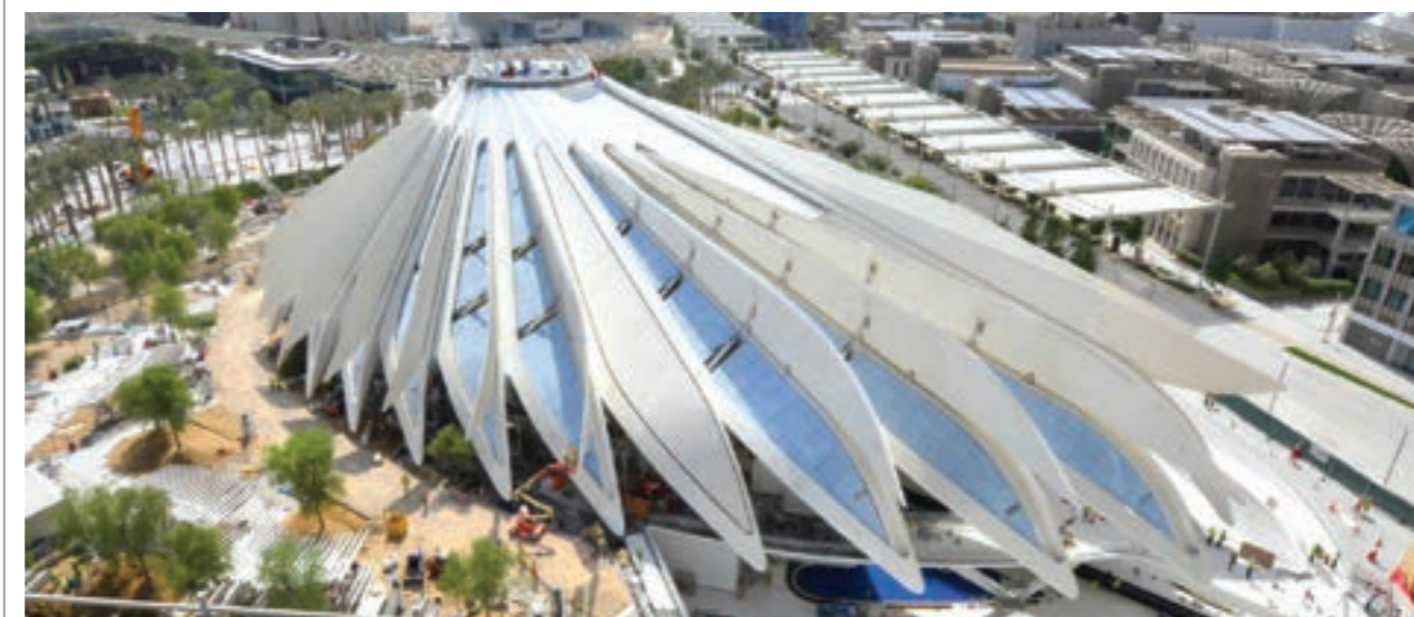
Figure (2): UAE Pavilion at Dubai Expo 2020 – Source: MOPA
